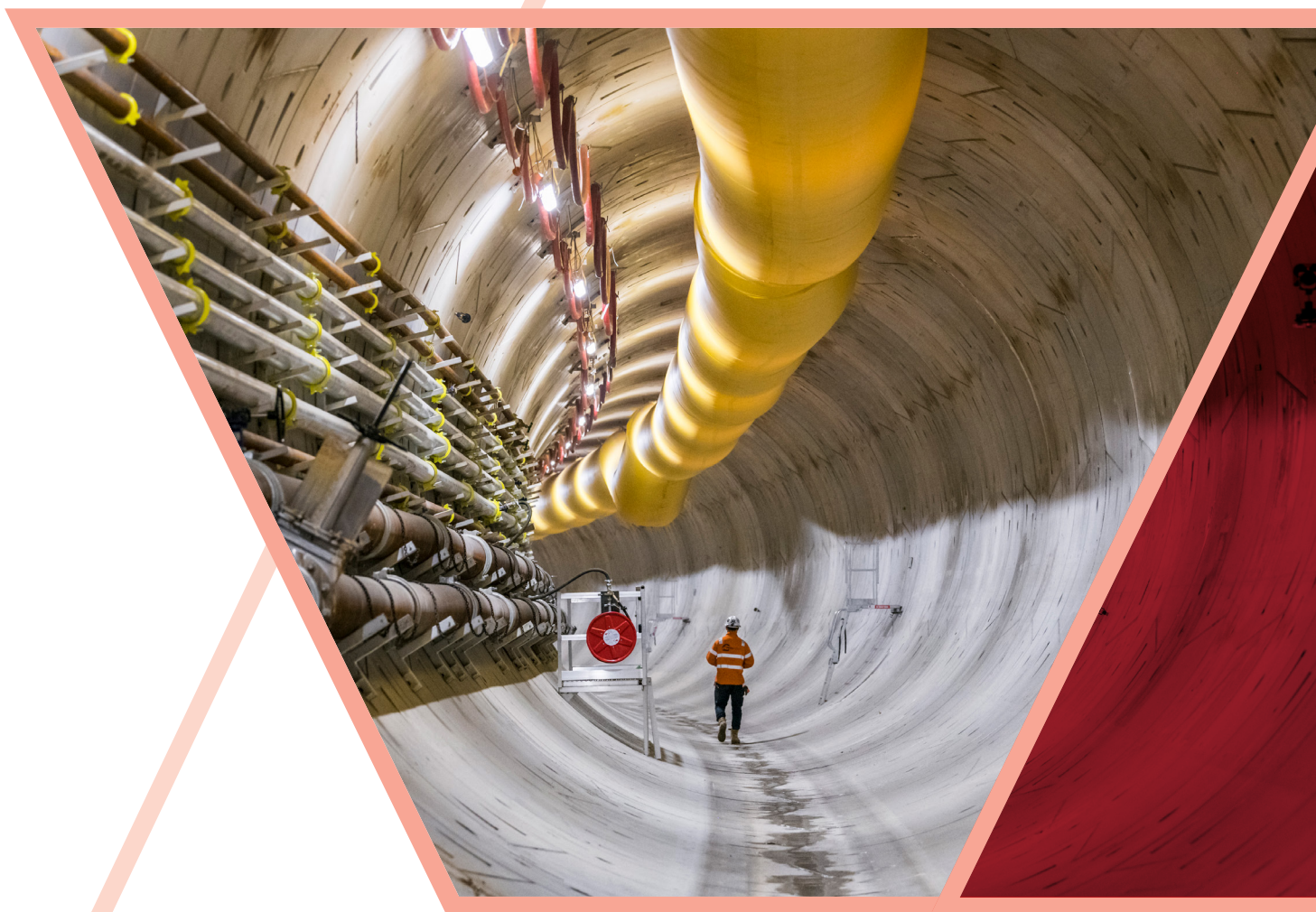
The Metro Tunnel Project – North Melbourne Tunnel.
