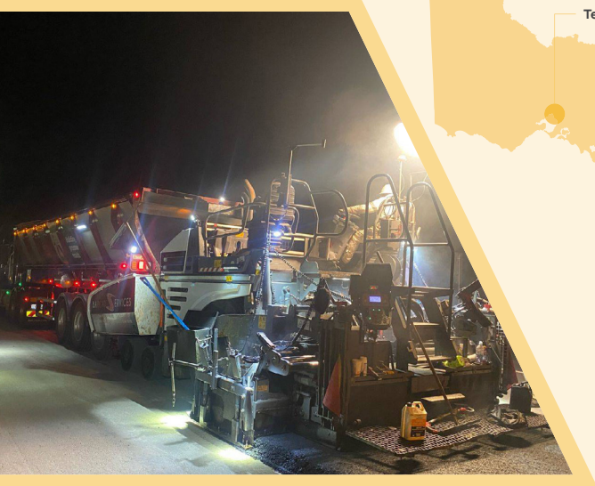
BA Road Services preparing a new road surface.
