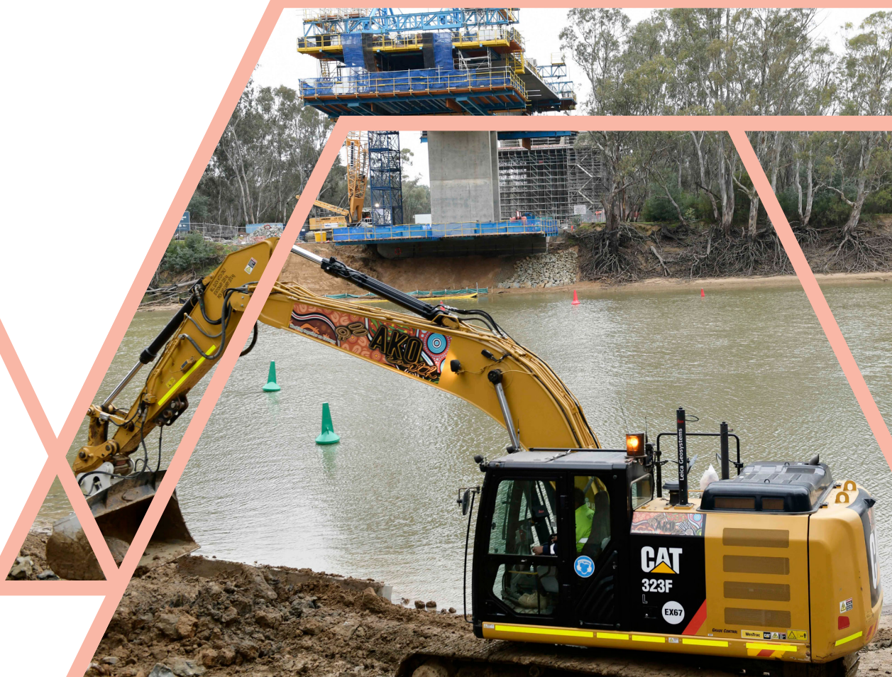
AKO Earth on site at the Echuca-Moama Bridge Project site.
