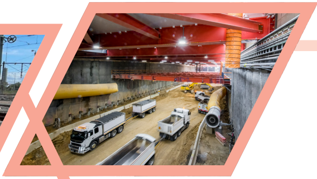
The Metro Tunnel Project – Parkville Station.
