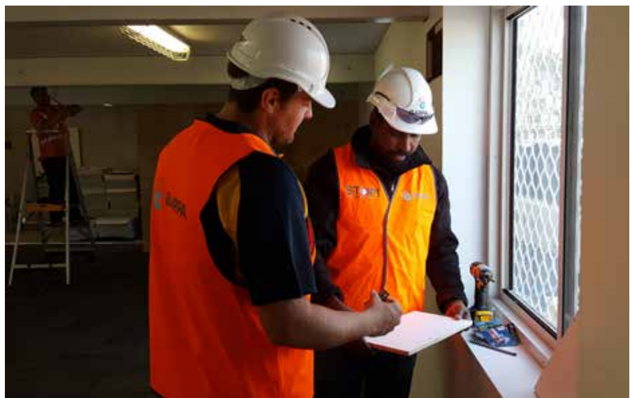
Barpa employees on site at the Mernda Rail Extension Project
