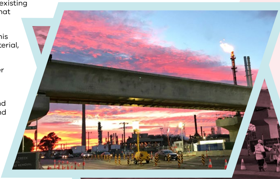
The Kororoit Creek Road Level Crossing Removal Project.
