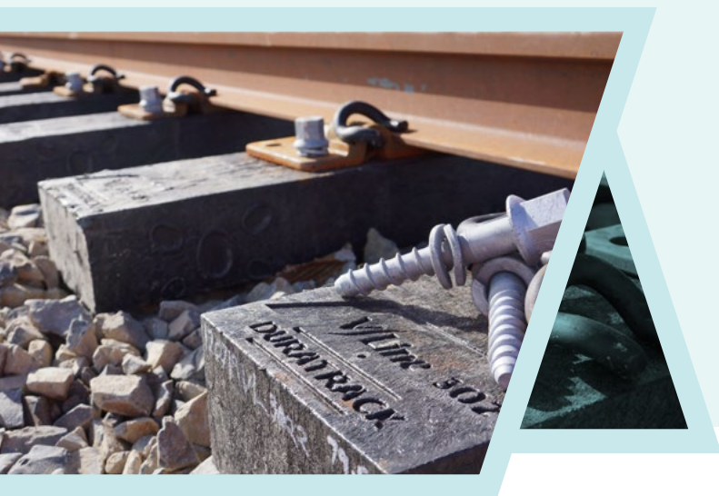
Recycled plastic sleepers at Wyndham Vale. Image: Level Crossing Removal Project.
